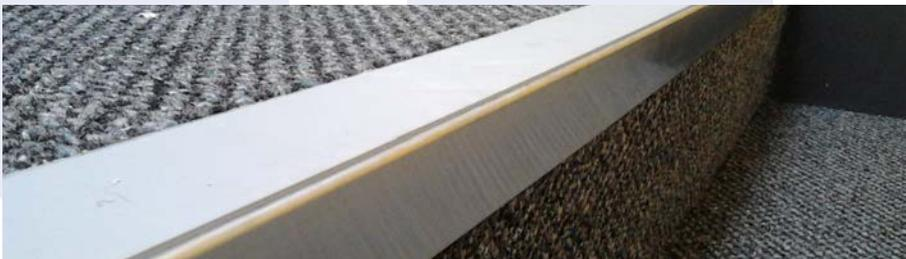
Quantum Flooring's specialist 'Secret Fixing' method of installation was used to ensure less risk of dirt traps forming also to securely hide all screw heads. This method of installation is quick which was important as the refurbishment had to be rapidly completed outside semesters in order to be ready for the 2013-14 academic year.
